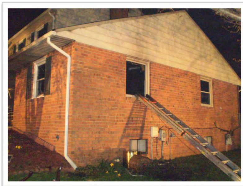
Figure 8: Side Delta showing the window, and the ladder placement where the fire fighter was removed.
