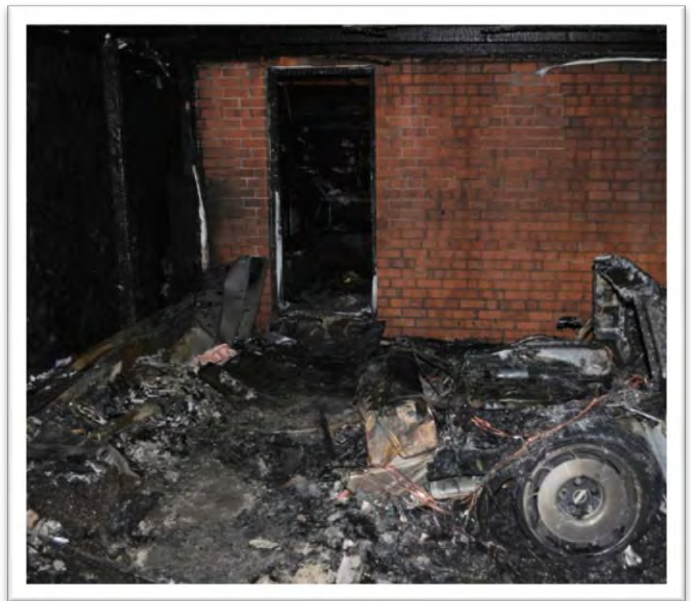
Figure 6: Side Bravo door leading from carport to interior of the structure.
