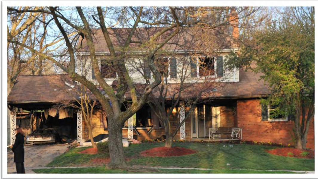
Figure 4: Side Alpha of the structure during daylight.
